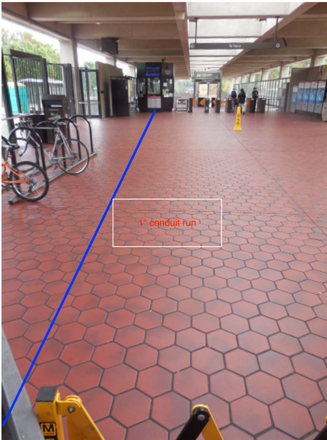
Photo #1 – F08 Southern Avenue: Duct run from Kiosk to AFC panel
